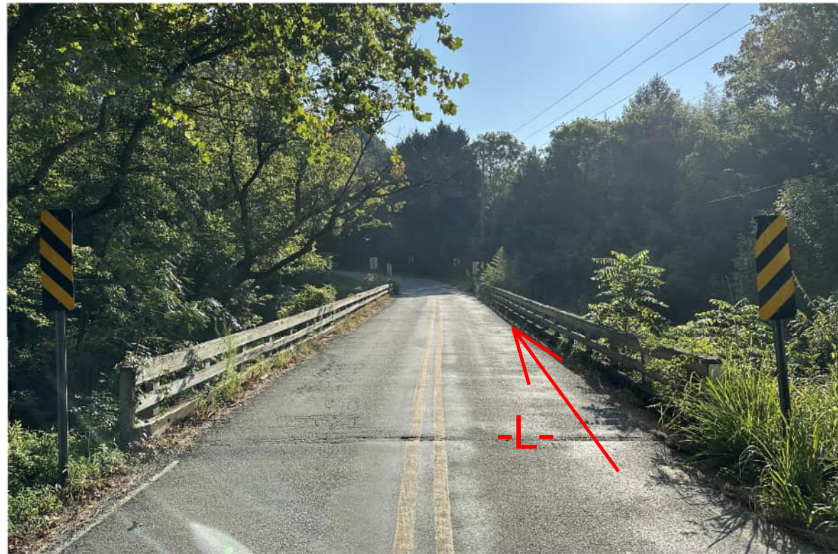
WEST APPROACH LOOKING EAST ALONG -L- ALIGNMENT
