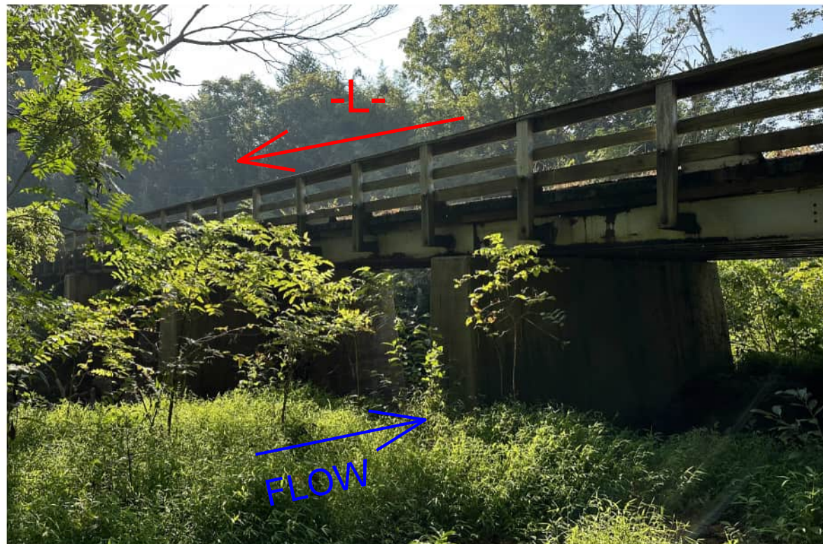
NORTH SIDE OF BRIDGE LOOKING SOUTH (DOWNSTREAM)
