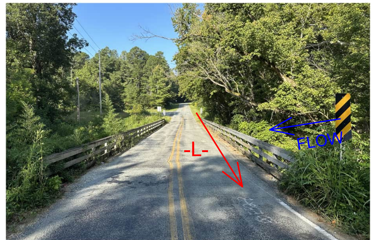
EAST APPROACH LOOKING WEST ALONG -L- ALIGNMENT
