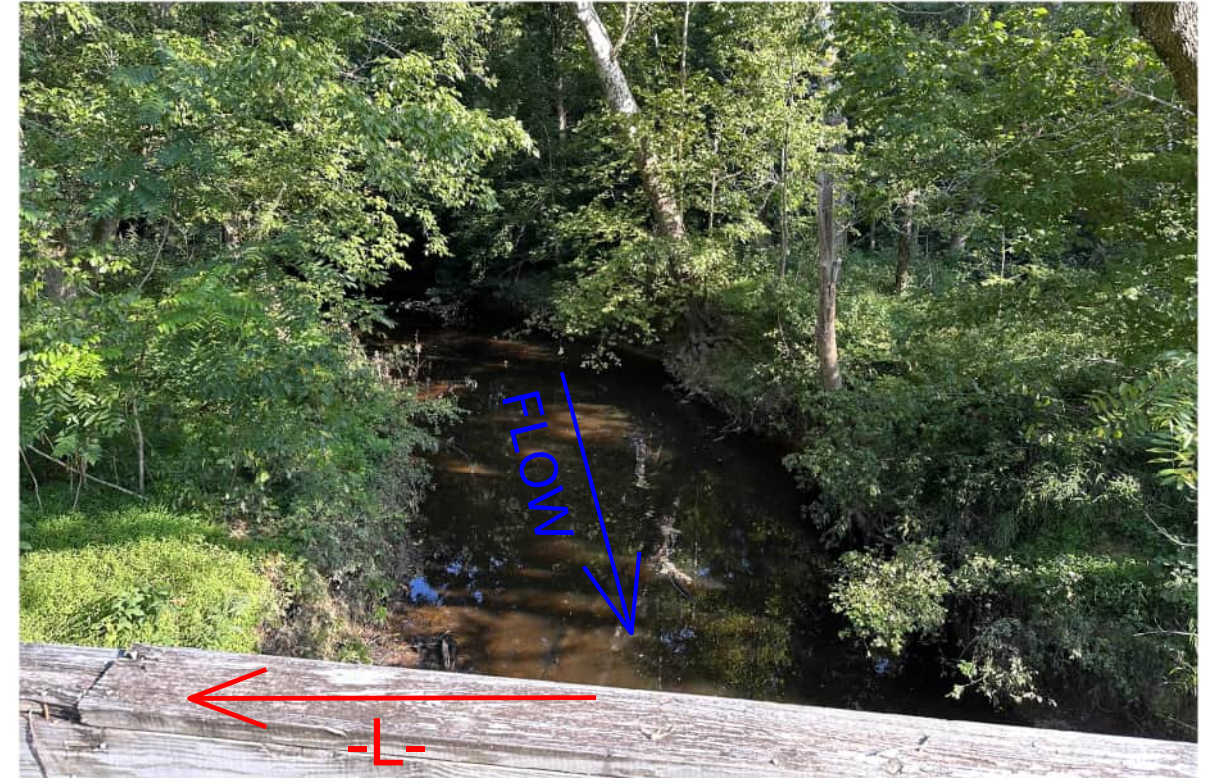
ON BRIDGE LOOKING NORTH (UPSTREAM)
